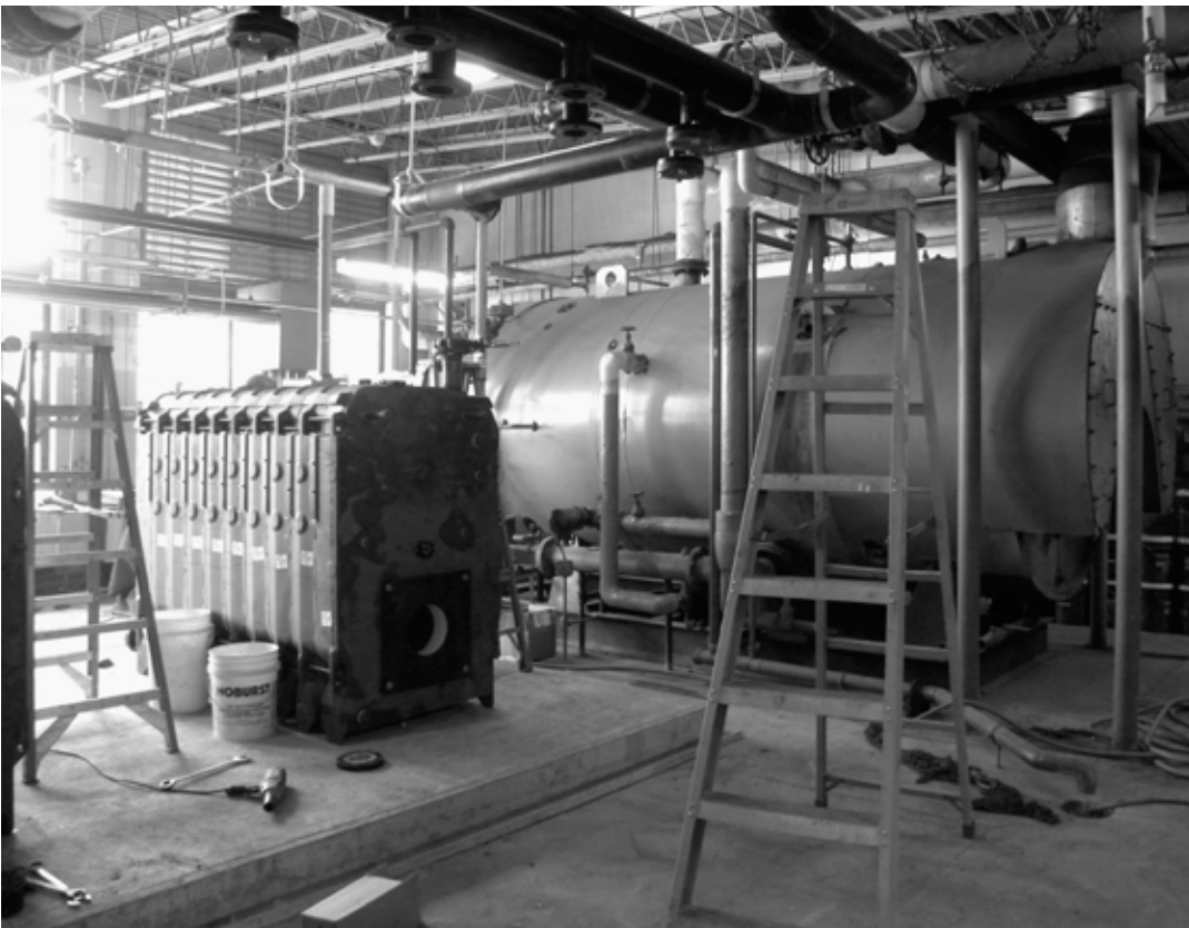
One new boiler, pictured on the left, was installed over winter break. The new boiler burns a better grade oil and much more efficiently than the old ones (right). Photo: Echo Staff
